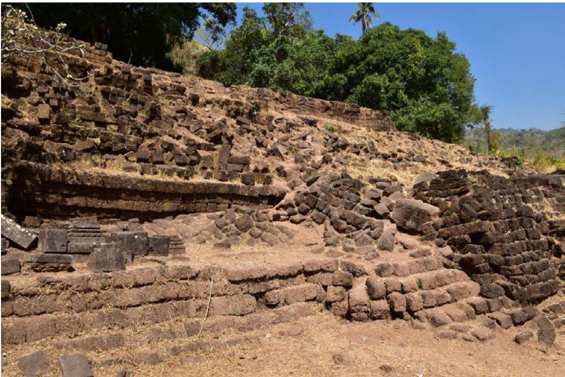
Fallen structures of 3 rd terrace
