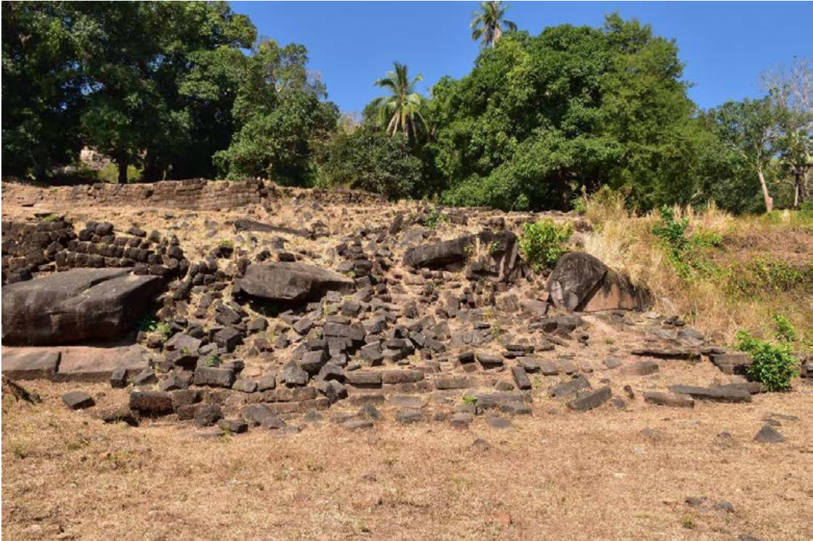
Fallen structures of 3 rd terrace
