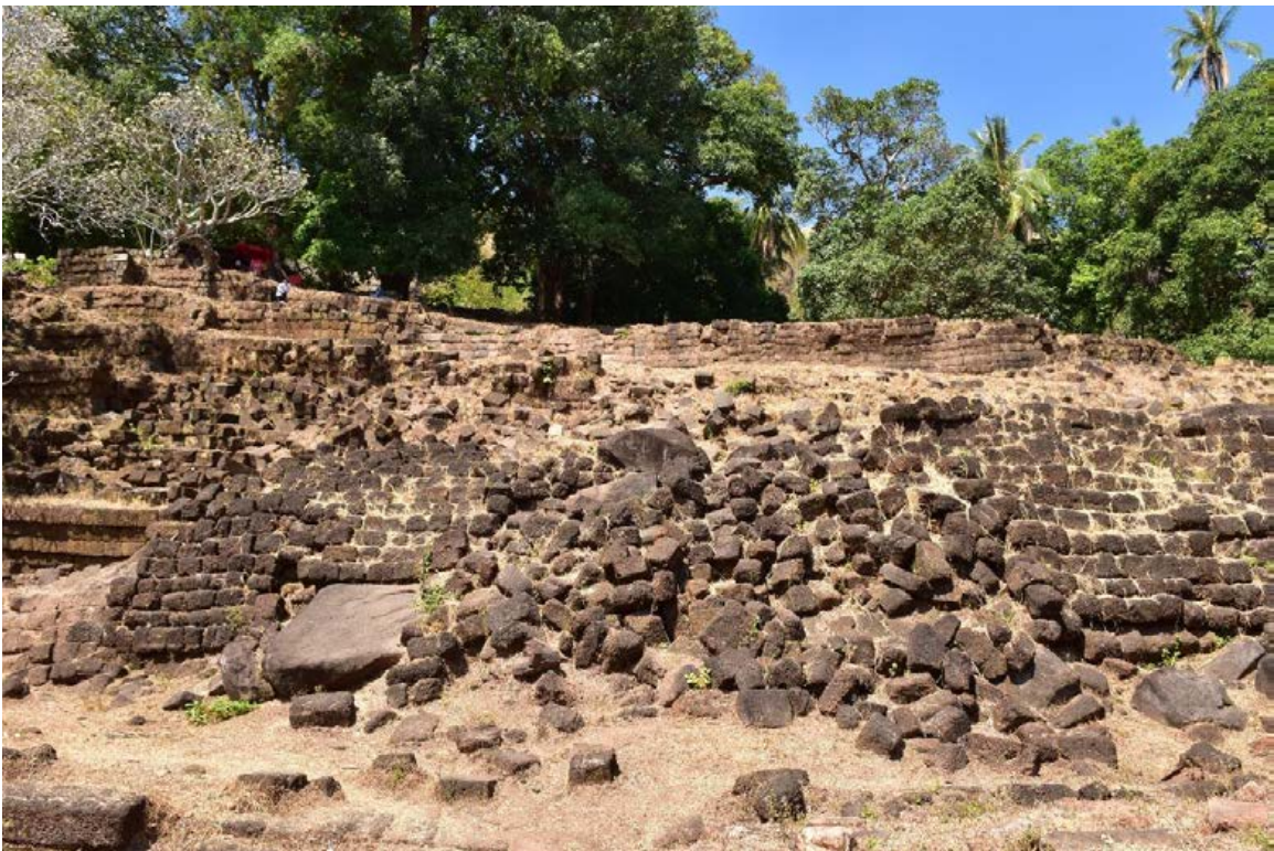
Fallen structures of 3 rd terrace
